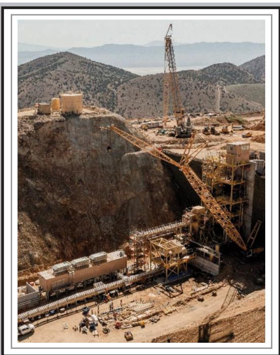
crusher now installed, construction of the new three-stage crushing circuit is now substantially complete. Once fully ramped-up, throughput is expected to average 32 million tons per year, which is approximately 2.5x higher than historical levels, making Rochester one of the world's largest open pit heap leach operations
